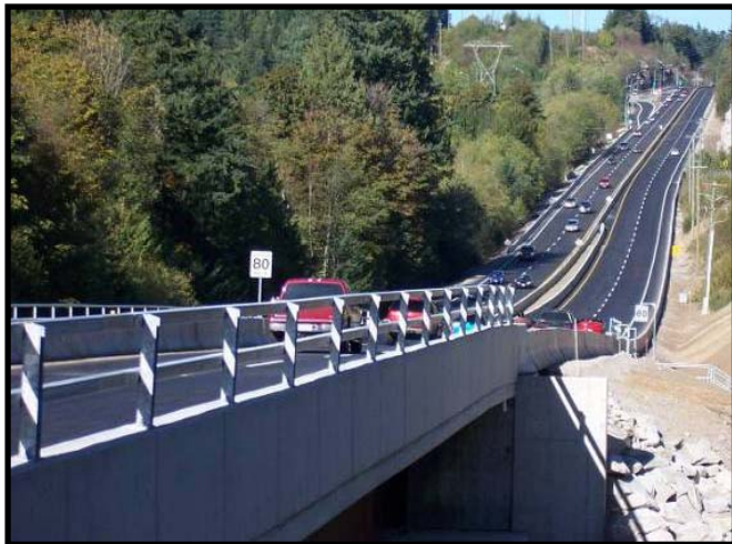
Sea-to-Sky Highway Improvement Project
